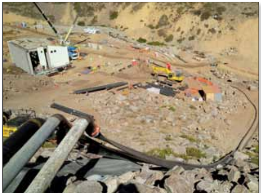
High pressure dewatering
