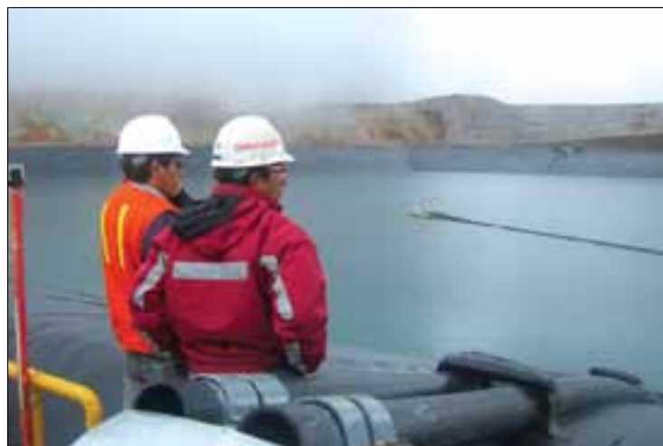
12" MINEFLEX on floating barge
