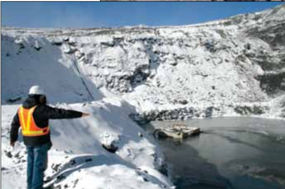
MINEFLEX in operation in sub-zero conditions
