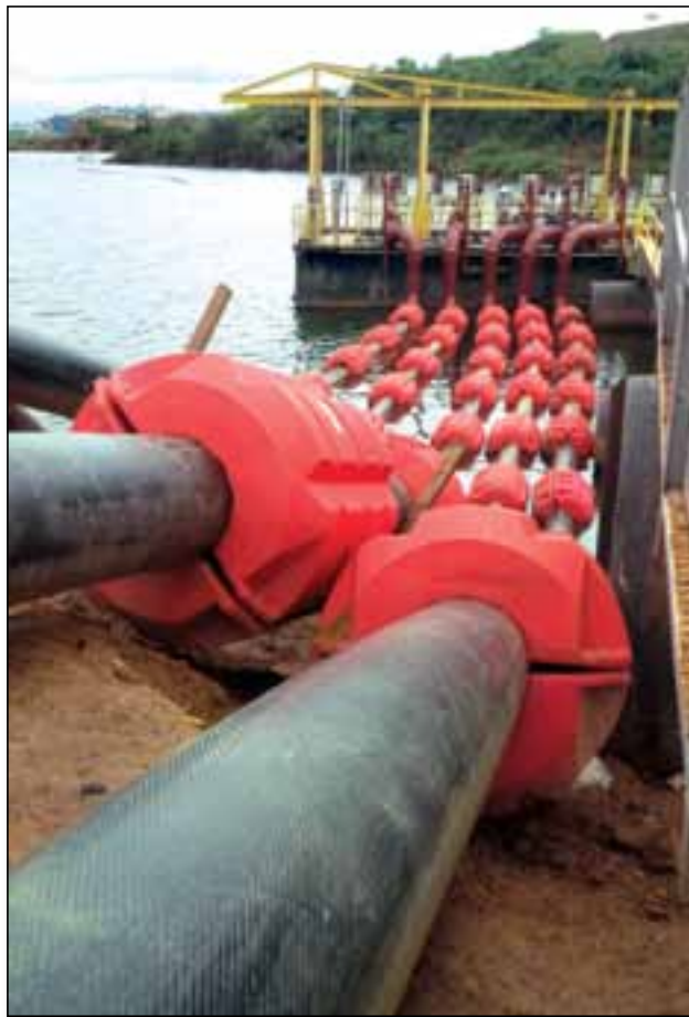
MINEFLEX on floating barge
